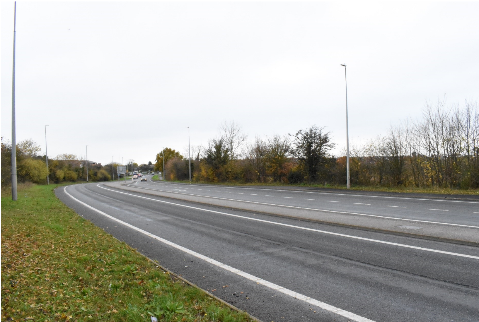
Plate 11: View of southern boundary of PDA from the former Thanet Way
